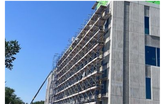
East elevation window caulking continues
