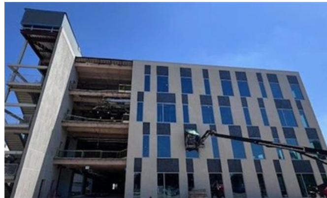
South elevation window caulking continues
