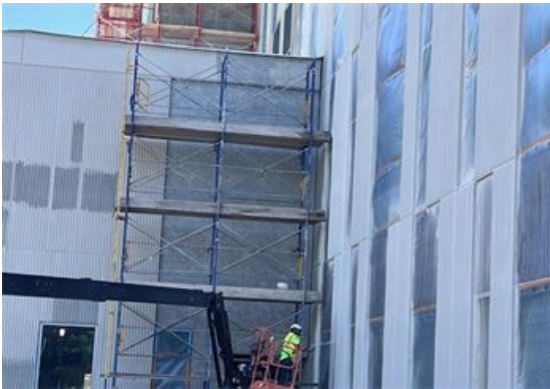
Exterior paint continues
