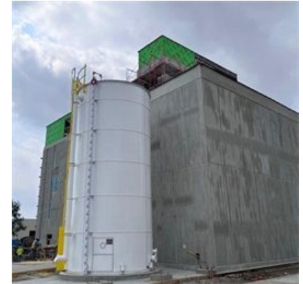
Fire Protection Storage Tank
